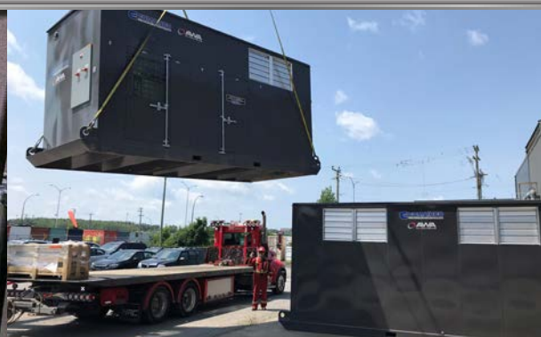
EASY HANDLING WITH LIFTING BRACKETS FOR CRANE
